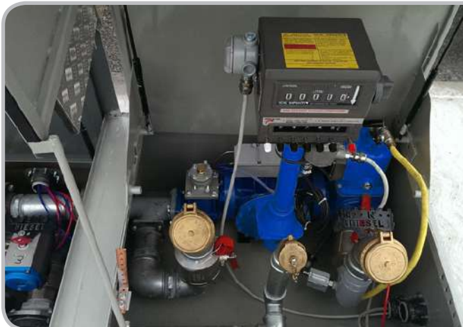
Drop/pressure download with AT04914 product quality sensor
